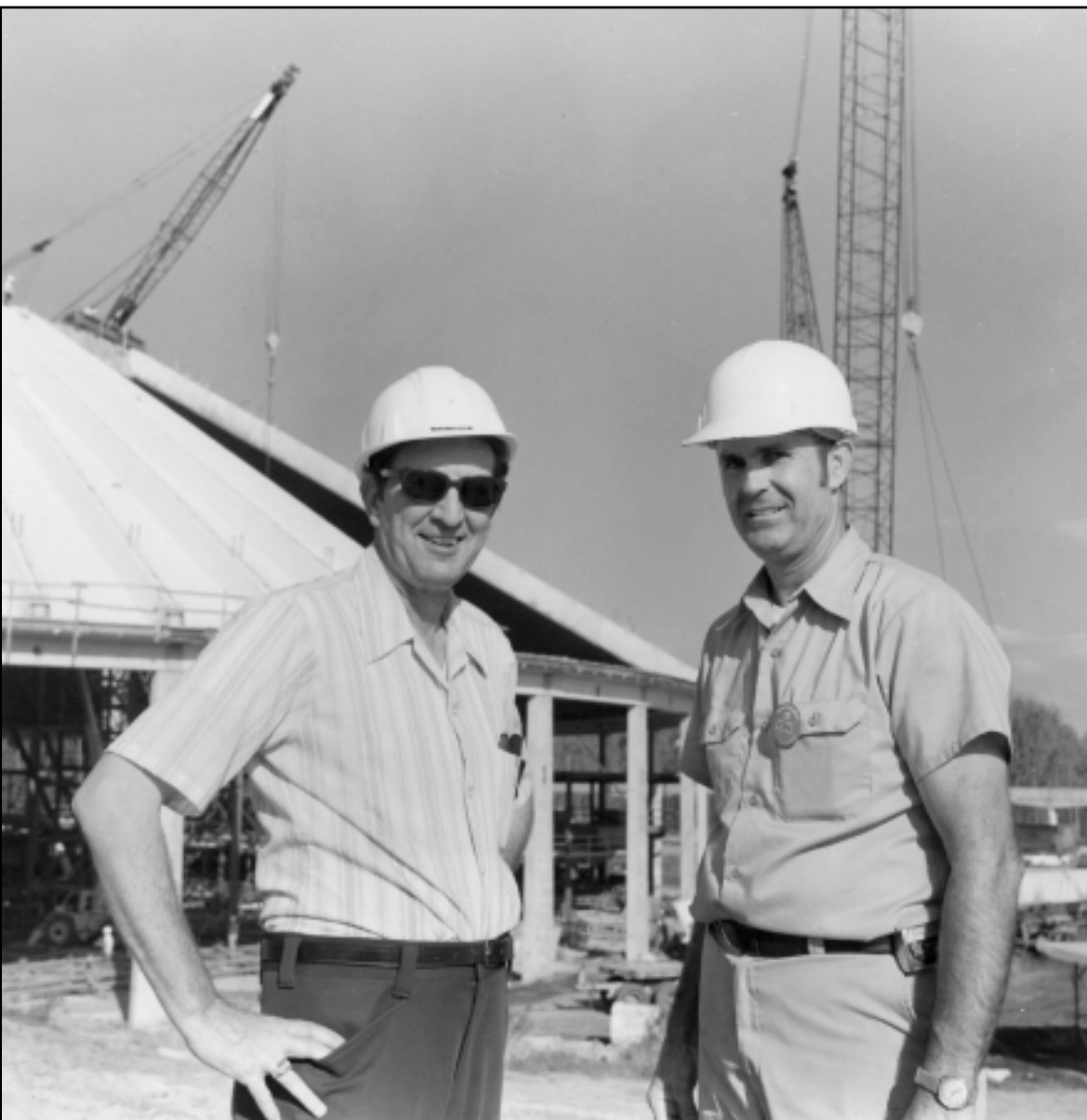
JOHNNY AYCOCK IS SHOWN, RIGHT, WITH BUDDY ADAMS. THE TWO MEN WERE VERY ACTIVE IN THE CONSTRUCTION OF SPACE MOUNTAIN AT WALT DISNEY WORLD IN ORLANDO, FLORIDA.
